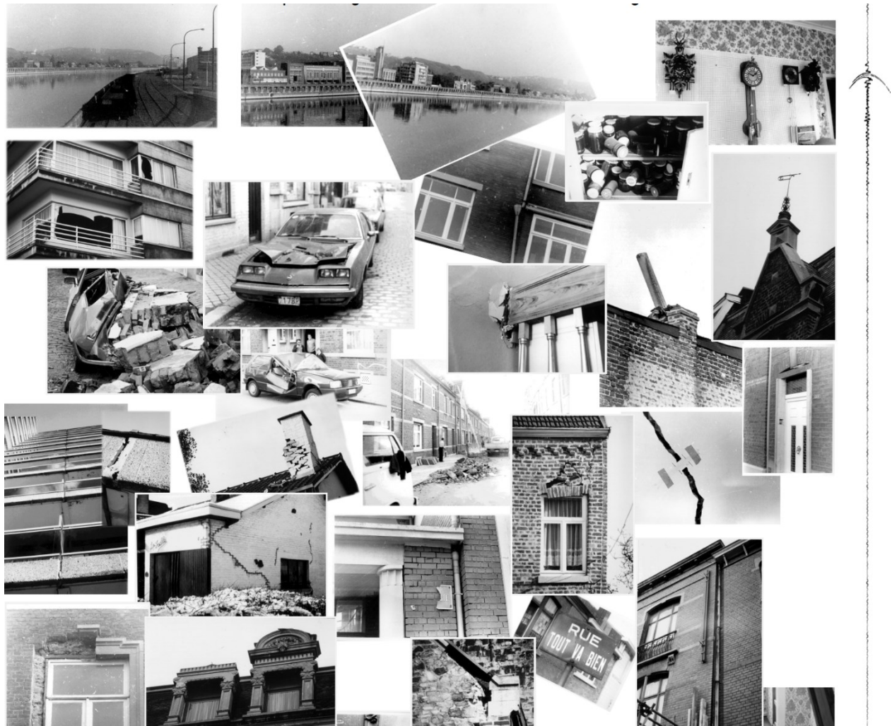
Figure 12: Pictures of damage in the epicentral area around Saint-Nicolas, Flémalle and Liège.
