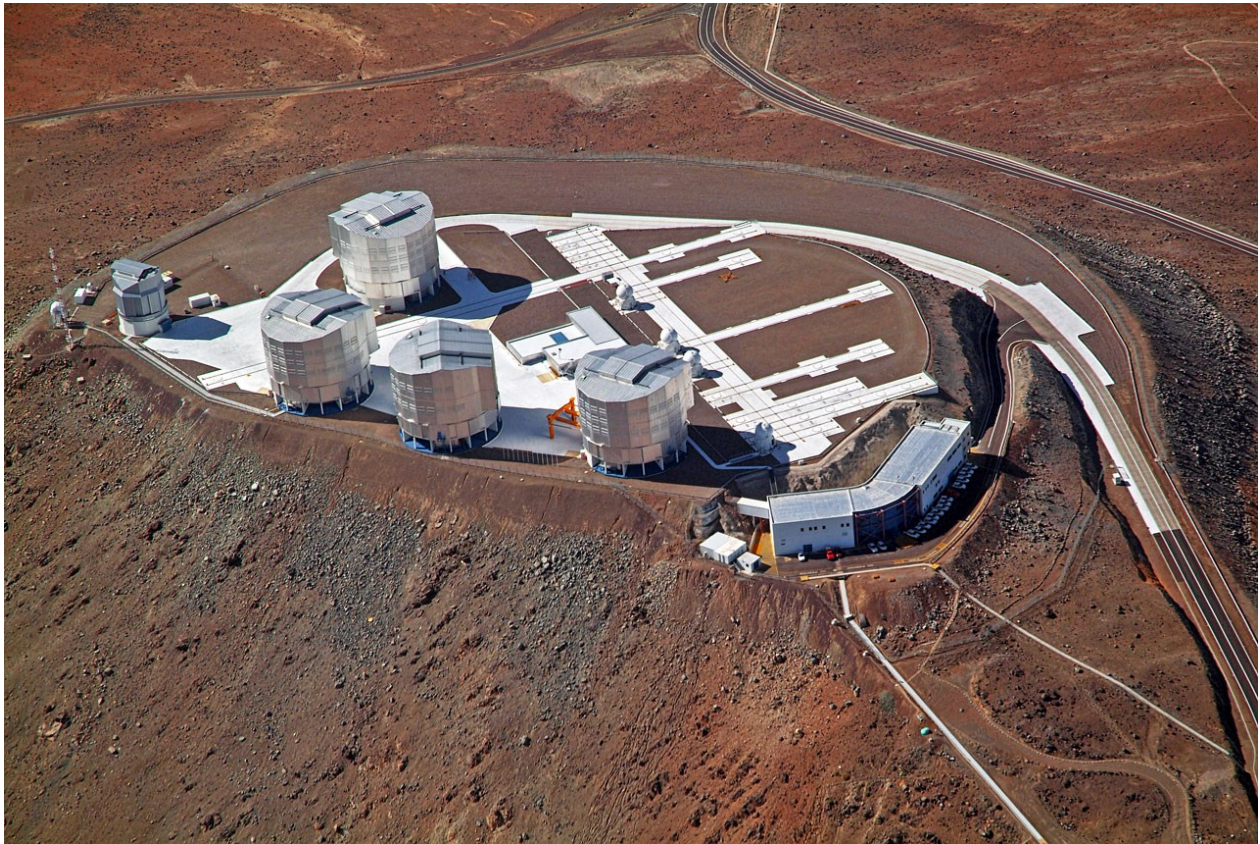
Figure 42: The Very Large Telescope (VLT) at Paranal, Chile. The Gaia-ESO Survey uses the Unit Telescope 2 (UT2), the second one from the right on the picture. This telescope has a multi-fibre instrument, called FLAMES, which can take about 130 spectra simultaneously. Credit: J.L. Dauvergne & G. Hüdepohl (atacamaphoto.com)/ESO.
